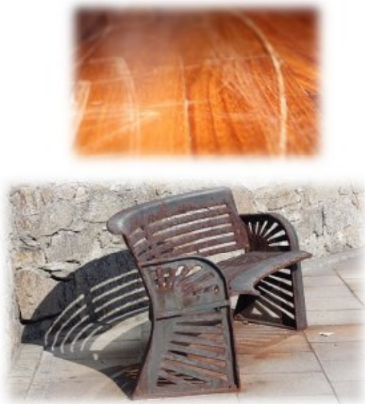
Fig.2: Scratches and corrosions that appear on surfaces.[7],[8]
