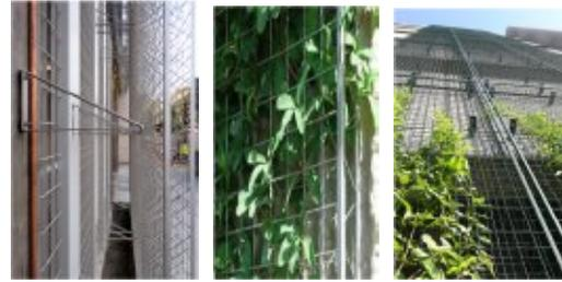
Figure (5) Wall mounted, modular three-dimensional panels, with standoff brackets, provide access to keep plants off the wall. Source: (15) [A North American Aluminum Industry Sustainability Report 2011].
