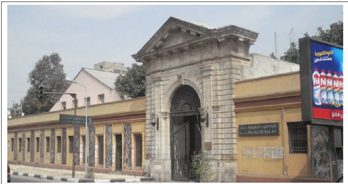
Figure 1. Faculty of Applied Arts main entrance.
